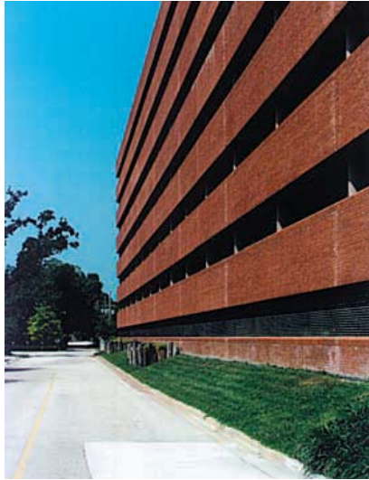
Parking Garage: Auto-Oriented Façade
