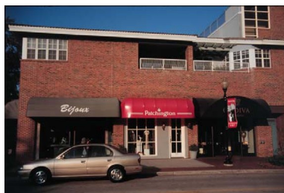
Retail shops on the street level with residential use above.
