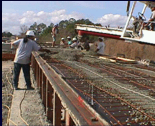
Parking garage construction at Florida Community College, Jacksonville.
